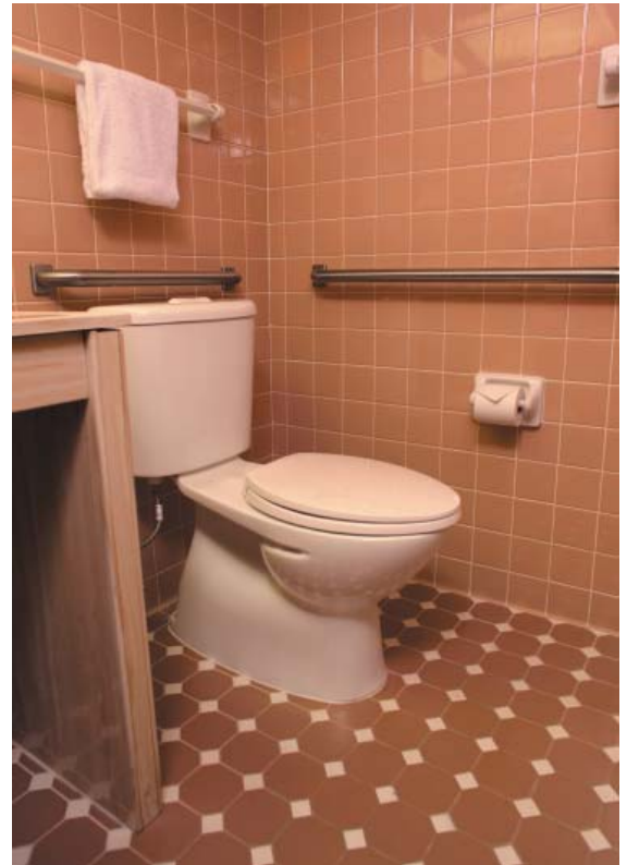
Image 1: Caroma toilet installation at Pear Tree Inn
