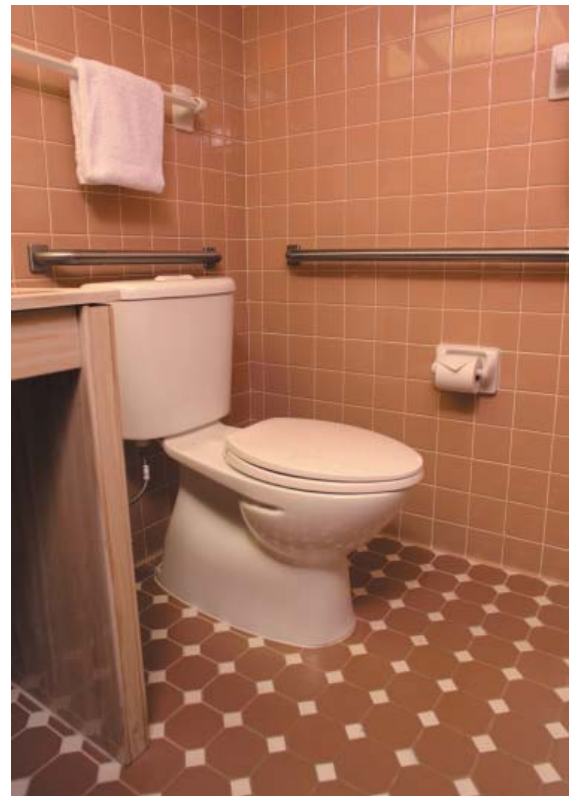
Image 1: Caroma toilet installation at Pear Tree Inn
